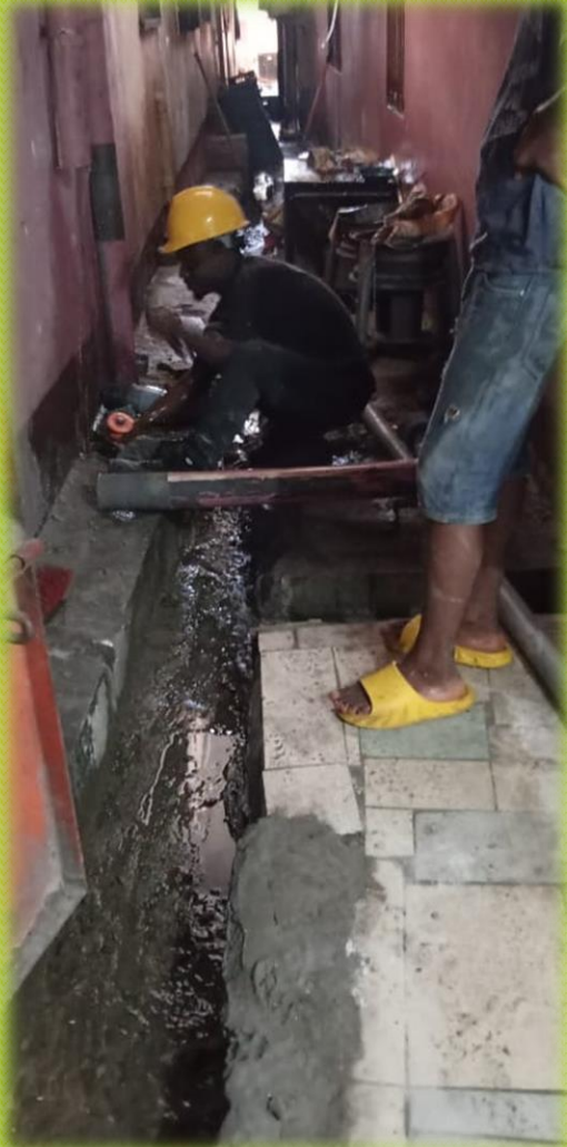
Aligning water drainage pipe
