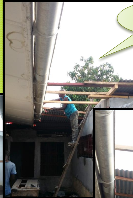
Courtyard Cover Prep
