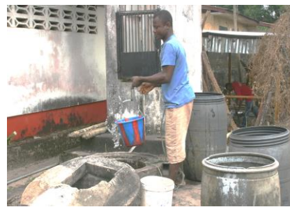
Water well for Agriculture needs to be capped for safety
